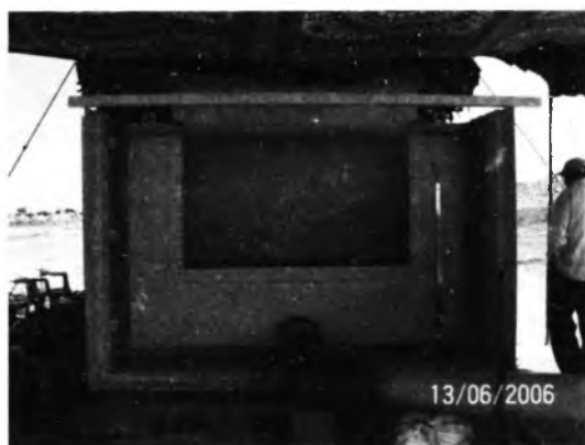
Photo 5 Surge pool arrangement
